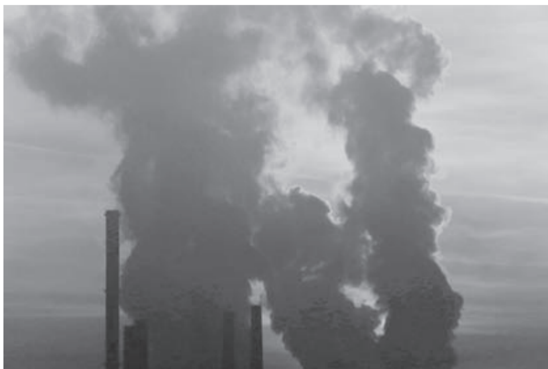
The sun sets behind a power plant powered by coal in the Bosnian town of Tuzla, 120 kms north of Sarajevo, Bosnia, Saturday, Dec. 12, 2015.
